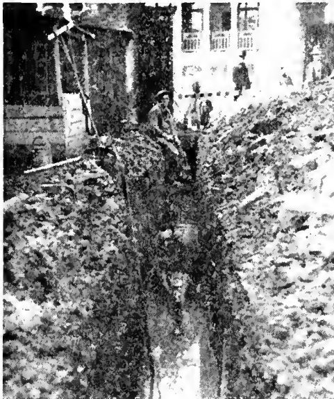
Refugees digging a sewer and drainage ditch
